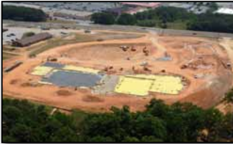
Beginning construction on Riverdale Town Center - 5% completion.
