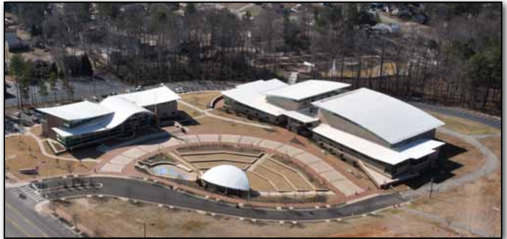
Riverdale Town Center project - 95% completion.
